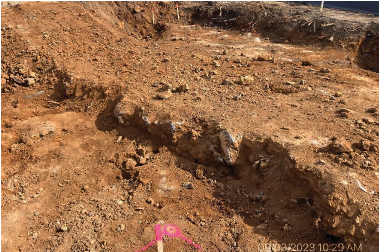
Figure 3. View south of pavement removal.
